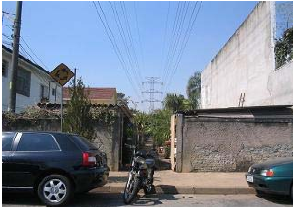
Figure 2 – Irregular construction close to a strip of servitude.
